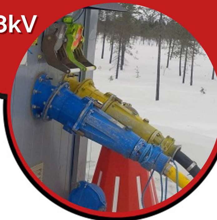
8kV, 400A Unshielded Couplers in service
